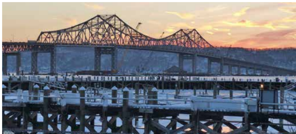
Bridge monitoring (Tappen Zee Bridge USA)
