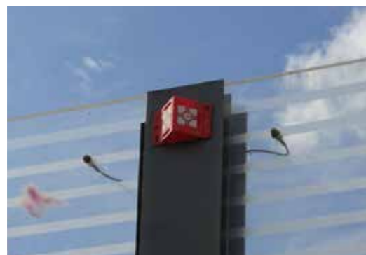
Observation of sound barrier walls.
