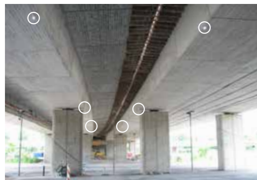
Observation of bridges.
