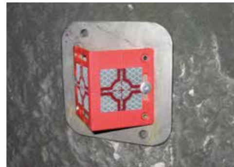
Coen Tunnel Amsterdam
