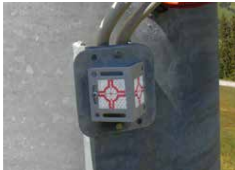
Survey point on the ski lift support
