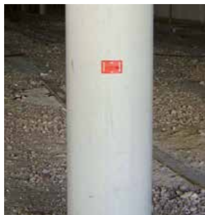
RS21r fixed to a column. The protrusion is cut in 4 – 5 times with a carpet knife.
