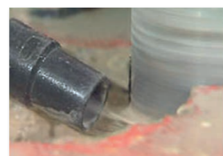
Vacuum drilling slurry
