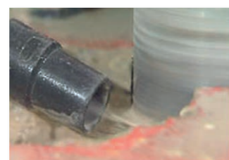
Vacuum drilling slurry
