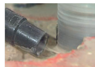
Vacuum drilling slurry
