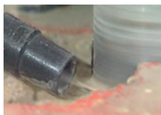
Filter outlet with drain gutter
