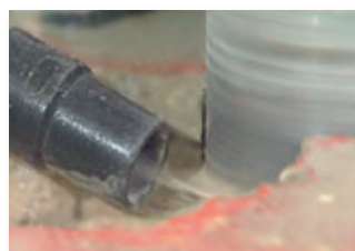
Vacuum drilling slurry
